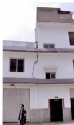
图 12 碰撞造成的破坏 Fig. 12 Damage caused by collision
