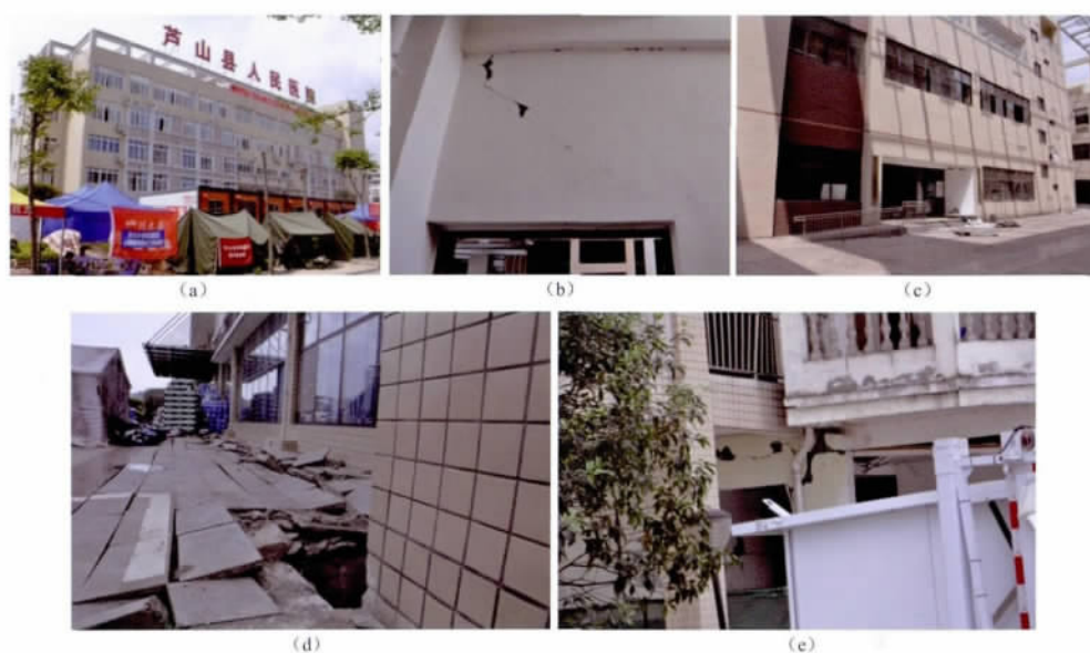
图 8 采用隔震结构的芦山医院在芦山地震中的表现. (a) 芦山医院全貌; (b) 填充墙轻微裂缝; (c) 医院对面芦山博物馆的震害; (d) 主楼与附属结构连接处的破坏; (e) 主楼与附楼连接处的破坏 Fig. 8 Seismic performance of isolated building. (a) Lushan Hospital; (b) Slight cracks on infill wall; (c) Damage of Lushan Museum opposite to Lushan Hospital; (d) Damage of connection between main building and attachment; (e) Damage of connection between main building and attached building
